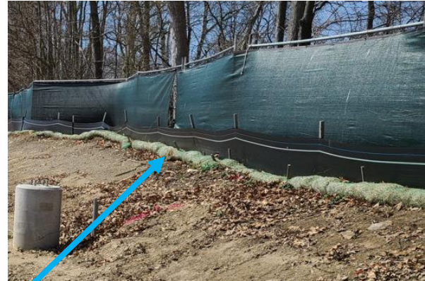
SILT FENCES AND WATTLES
