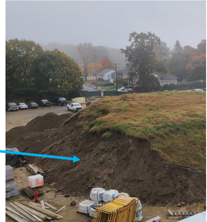
SEEDING EXPOSED CUTS/ STOCKPILES
