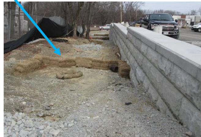
CHECK DAMS/ TEMPORARY SWALES
