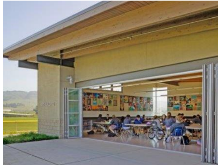
Connected to Classrooms
