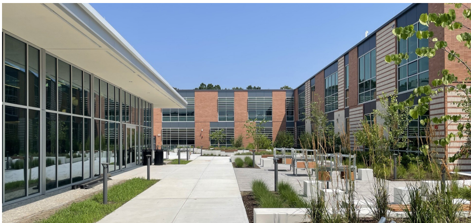
Construction Photo - Courtyard & Outdoor Classroom
